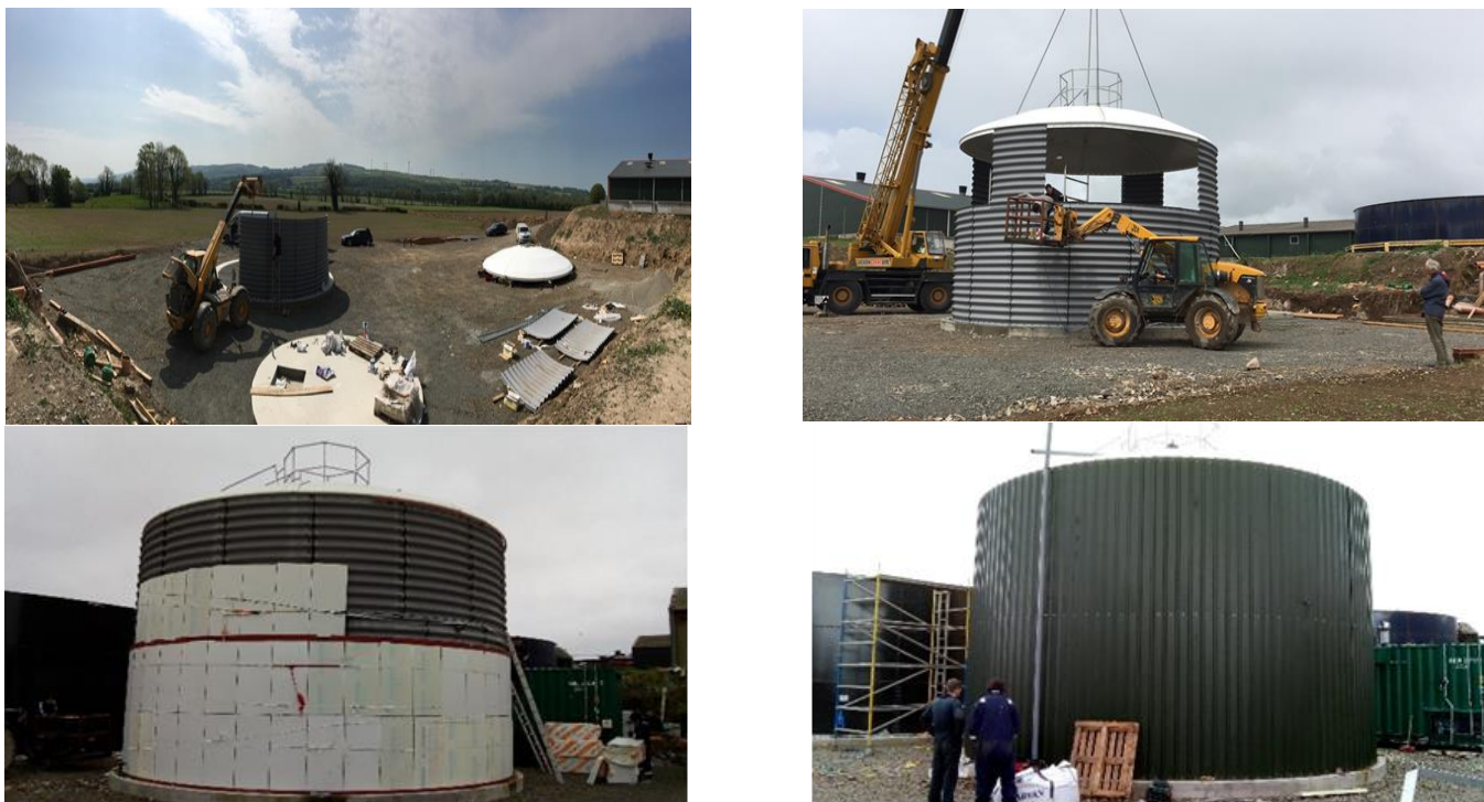
Figure5. Construction work of AD biogas facility at Ashleigh farms
