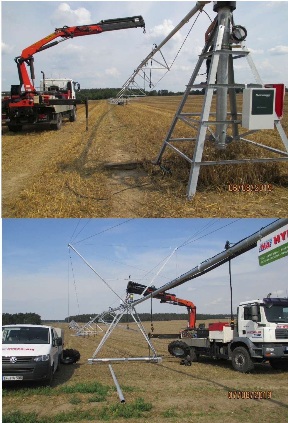
Figure 24 installation of the last tower and overhang stabilization
