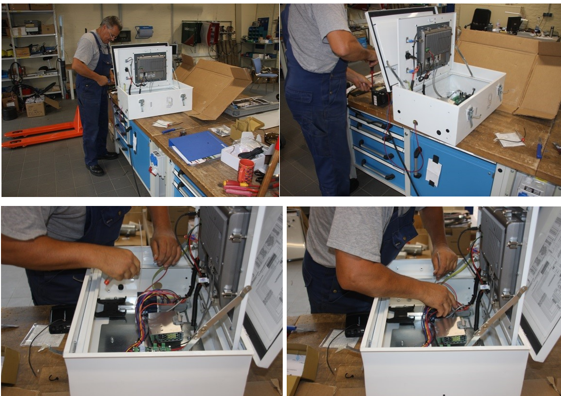
Figure 15 Wiring of the irrigation system
