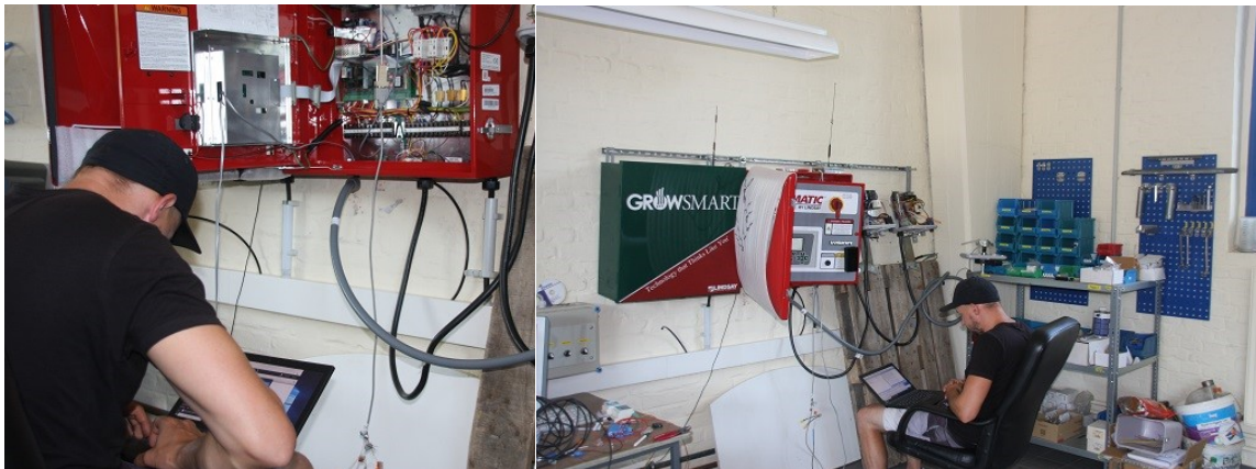
Figure 18 Reprogramming of the main controller
