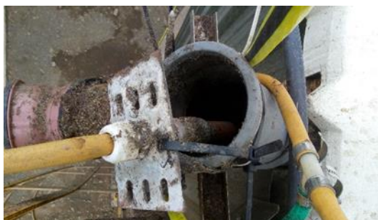
Figure 3. left image is the water-jet system in place, the right image is the simple water-timer to operate the jet every four hours.
