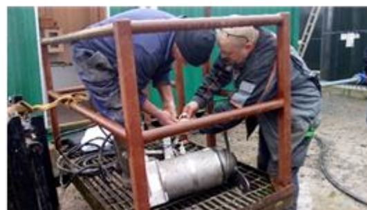
Figure 2. left image is compacted solids existing the pipework of the buffer tank, the right image is the sub-agitator ready for installation.
