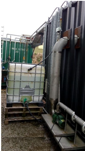
Figure 9. IBC plumbed with a ballcock to main water supply and outlet connected directly to flushing pump in biowave container.
